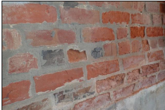
Masonry deterioration
