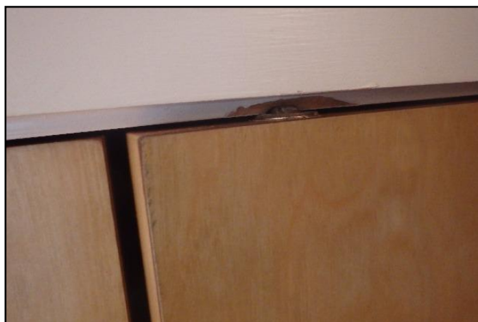
Does not latch properly
