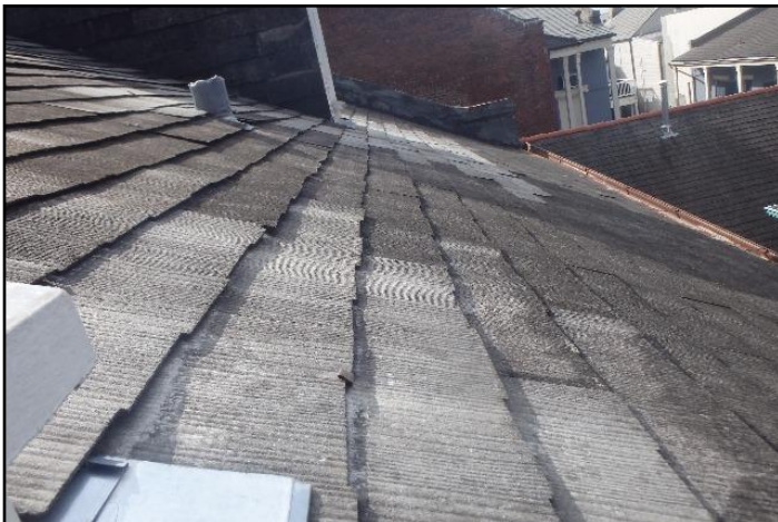
Fiber cement shingles
