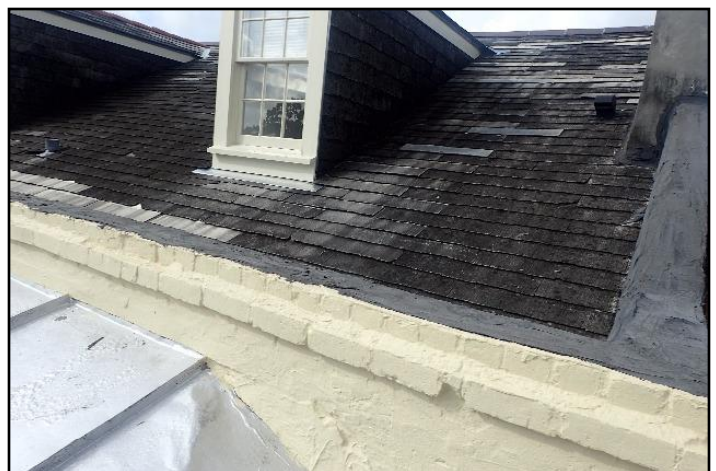
Fiber cement shingles
