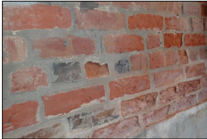
Masonry deterioration
