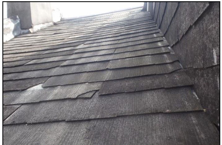
Fiber cement shingles
