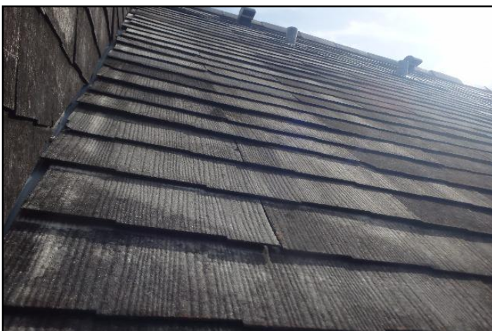
Fiber cement shingles
