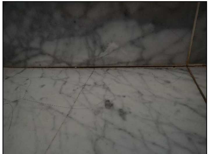
Grout loose, missing or deteriorated
