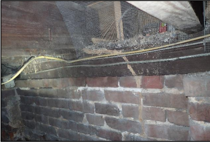
Mortar deterioration
