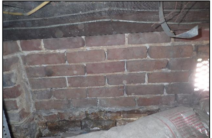
Mortar deterioration
