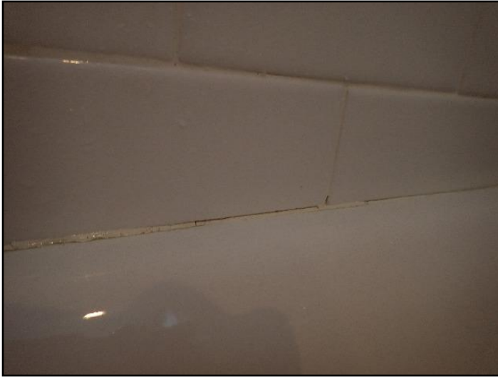
Grout loose, missing or deteriorated
