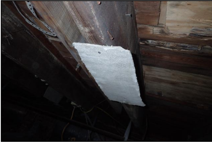
Suspect material- Furnace heat shield...
