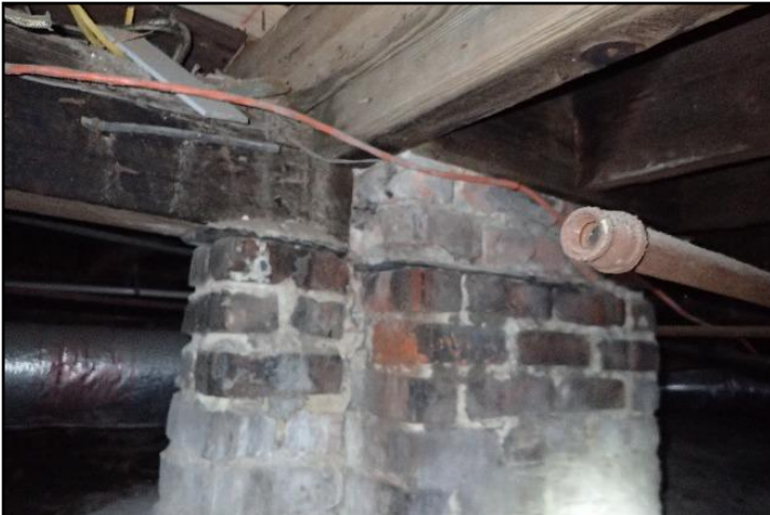
Mortar deterioration
