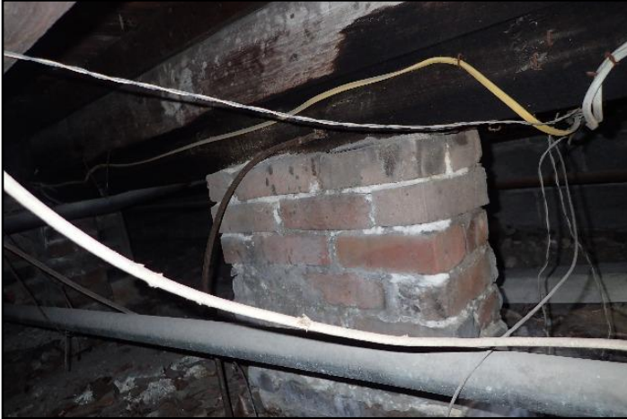
Mortar deterioration
