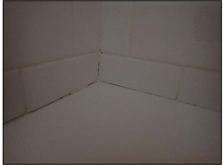
Grout loose, missing or deteriorated
