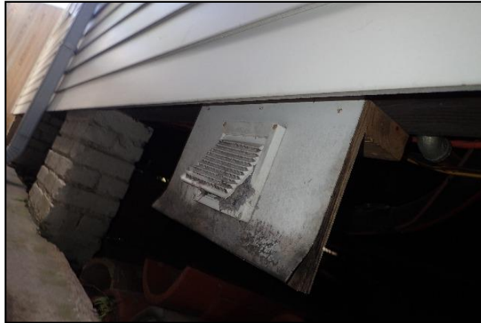
Dryer exhaust vent clogged with lint.
