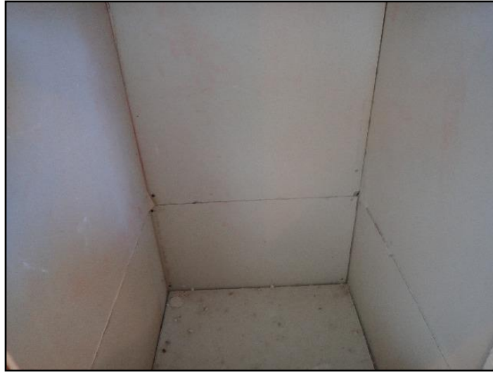
Return air chase unfinished with drywall or...
