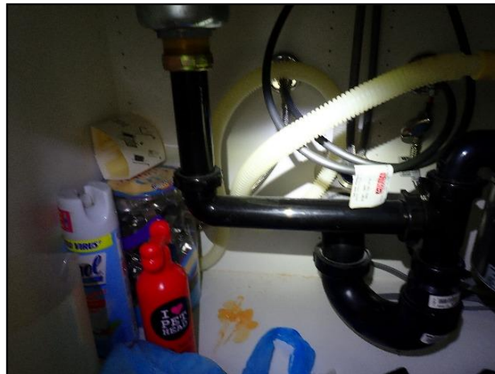
Backflow prevention missing
