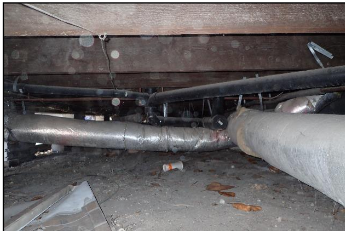
HVAC duct limited the inspection of the...
