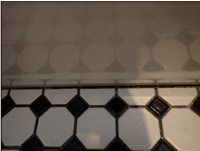
Grout loose, missing or deteriorated
