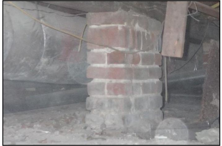
Mortar deterioration
