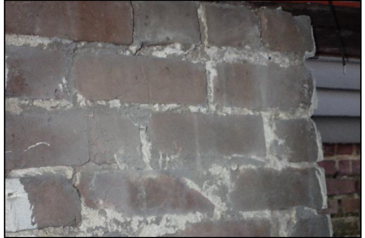
Mortar deterioration
