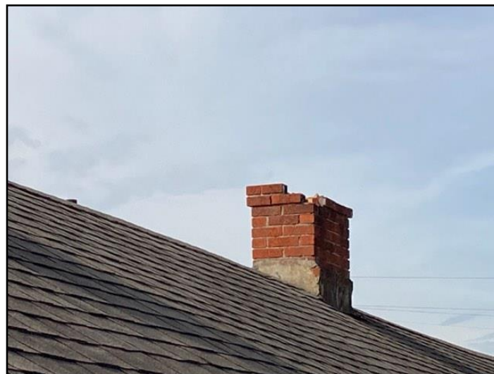
Loose, missing or deteriorated masonry
