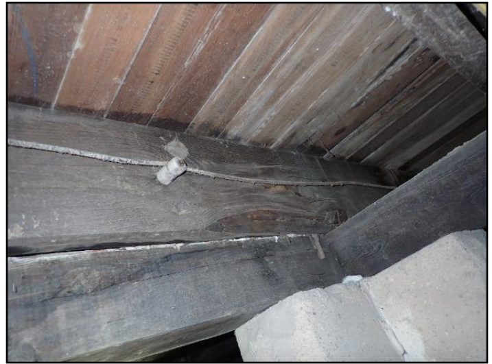
Inactive knob and tube wires found
