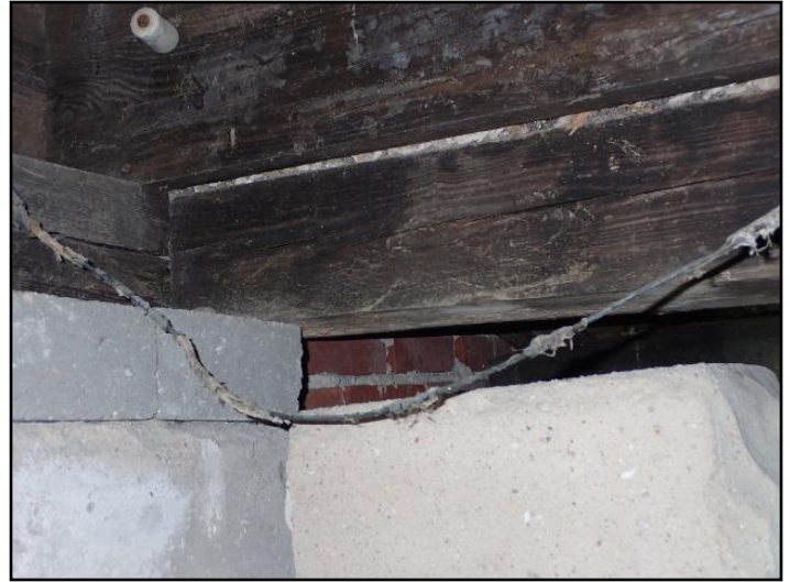
Poor end bearing on pier.
