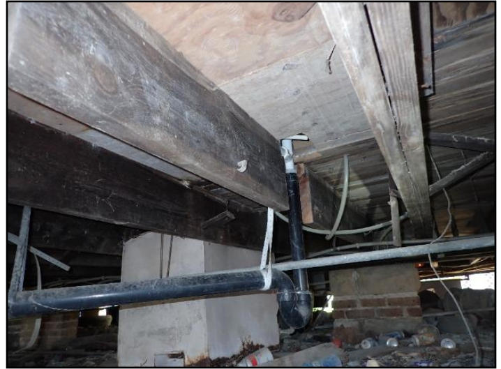
Cut joists
