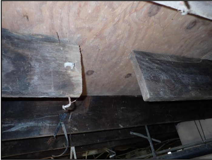
Cut joists
