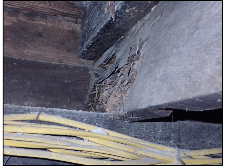
Rot and/or insect damage
