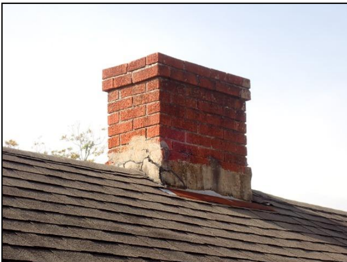
Metal flashing not visible
