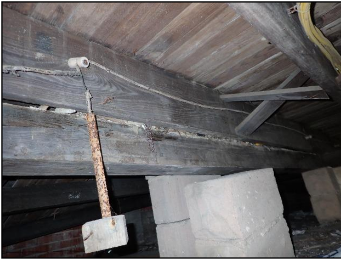
Inactive knob and tube wires found
