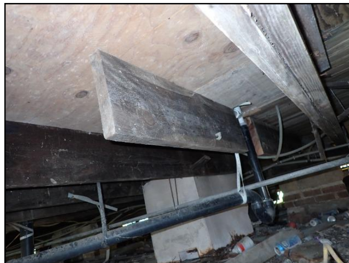
Cut joists
