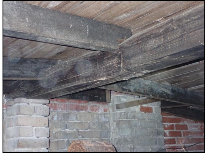
Form boards not removed
