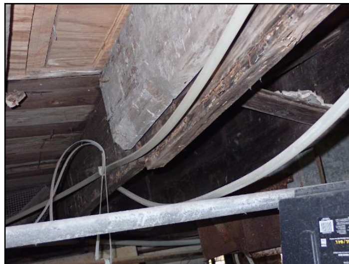
Rot and/or insect damage
