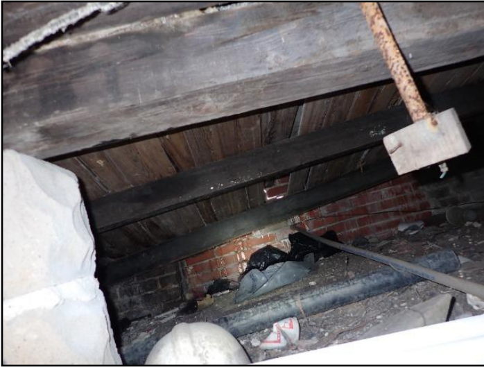
Form boards not removed
