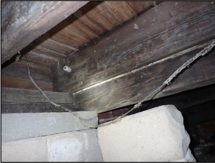
Poor end bearing on pier.
