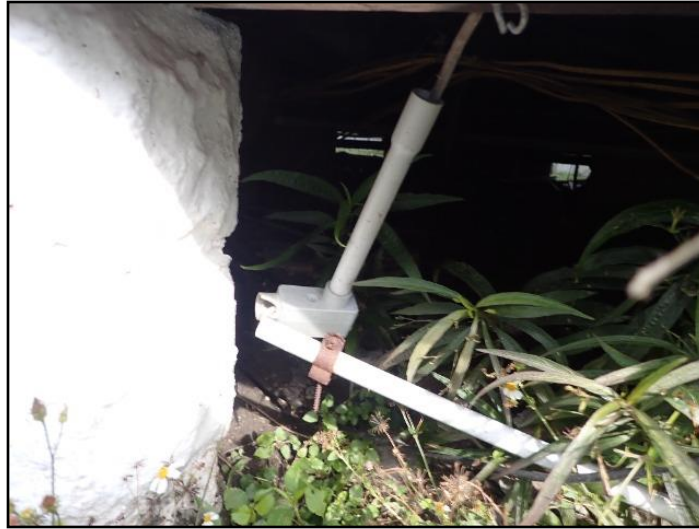
Damaged, missing, or corroded conduit
