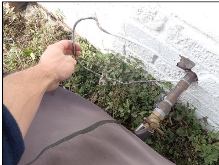
Disconnected ground wire
